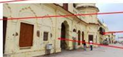
GANGA MAHAL: WINDOW, ARCH, PILASTER, PARAPET & CORNICE
